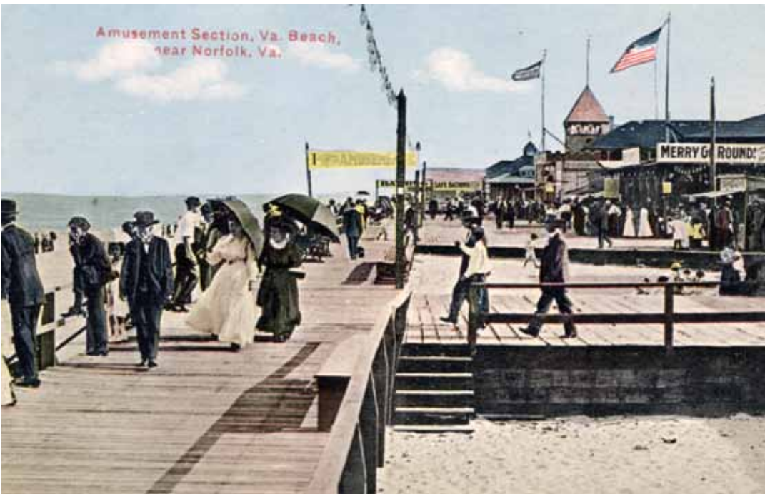
View of Virginia Beach boardwalk and amusement area, circa 1910. Borrelli would operate a carousel here with Dolle’s widow, Elizabeth.
